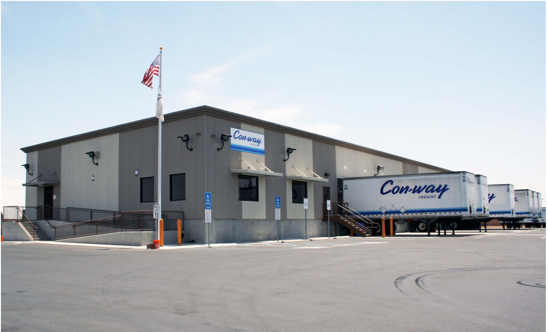
Conway Freight / Calexico, CA 10,000 sf Commercial warehouse and service center
