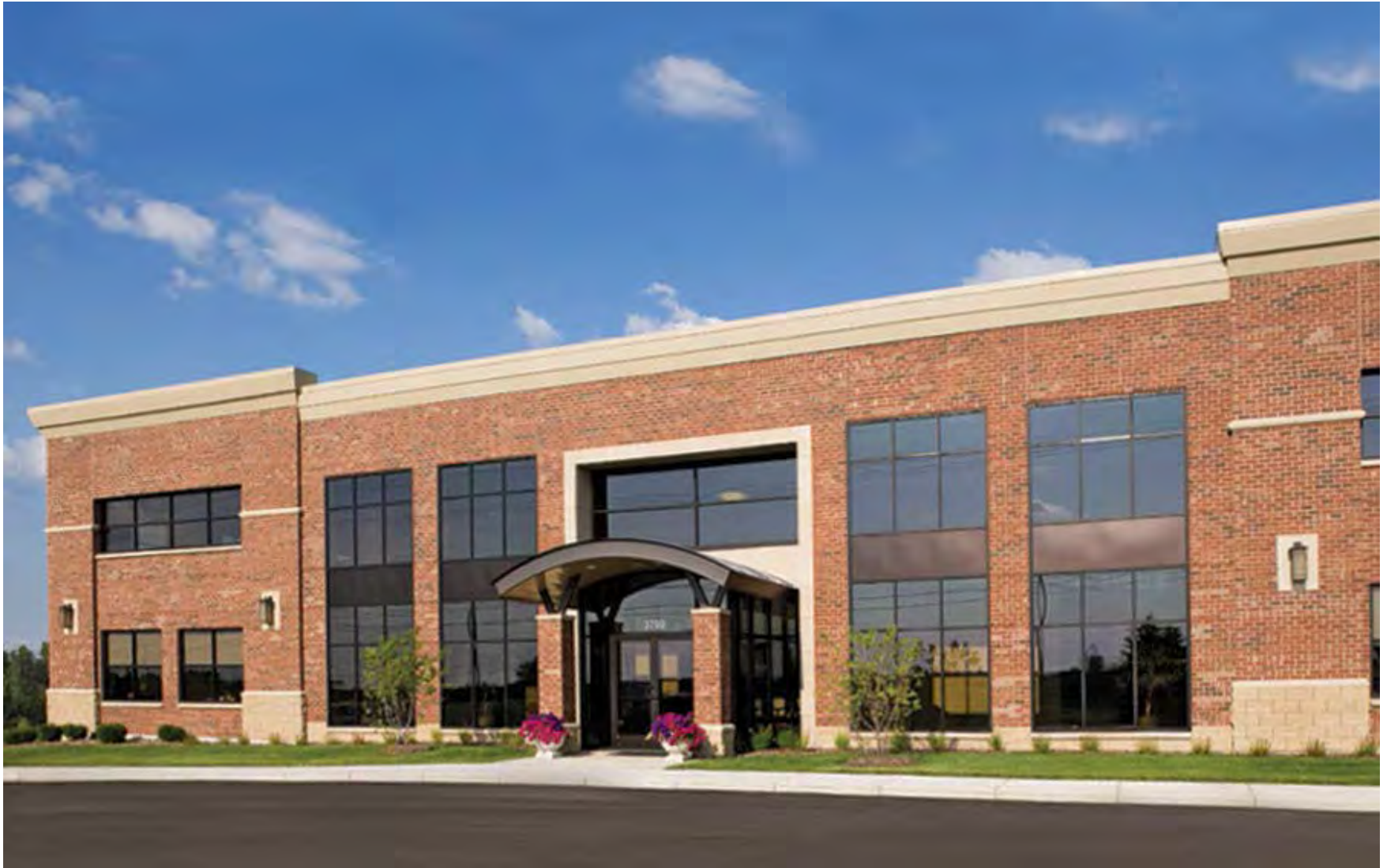
Action Fabricators, Kentwood, MI 66,440 sf manufacturing facility
