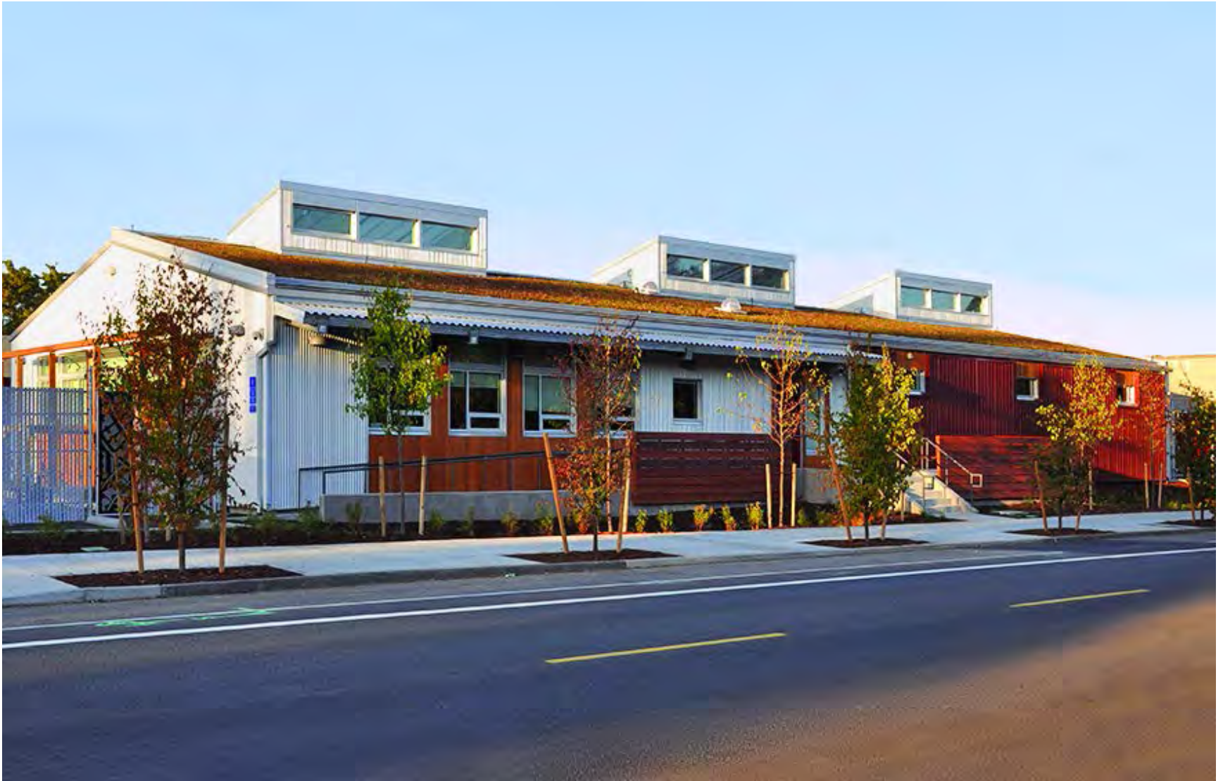
Flavel Maintenance Building / Portland, OR 7,000 sf Maintenance facility features living green roof
