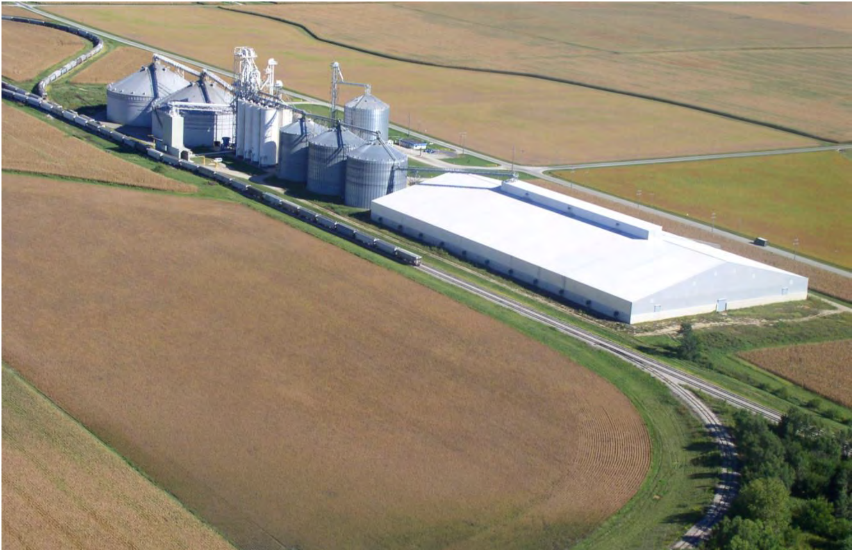
Fairbury Elevators / Pontiac, IL 226,500 sf Grain storage building
